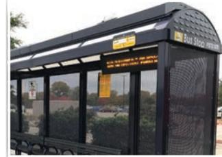
Roof houses batteries, energy management system and data communications
